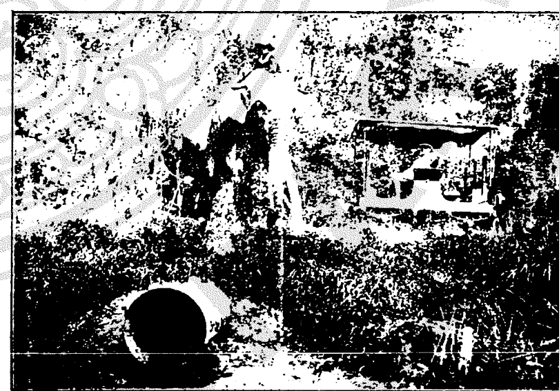
3' Dia. Armco Iron Nestable Culvert 32' Long at Ban Dan.
