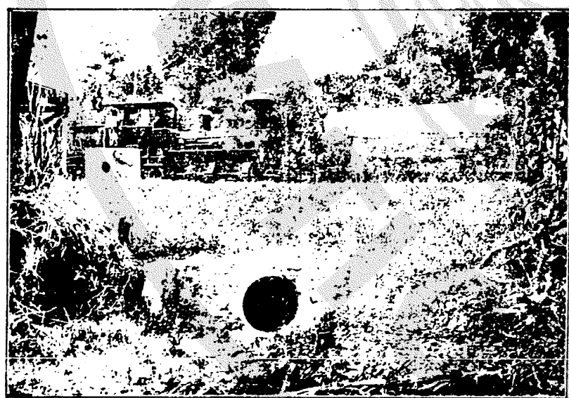
5' Dia. Armco Iron Nestable Culvert 65' Long at Nong Nam Kiew.
