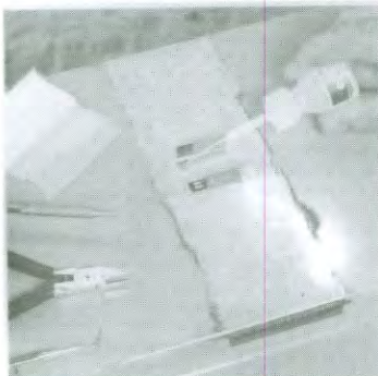
4. Applying the adhesive
