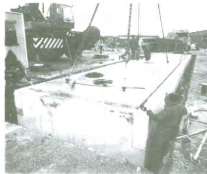
Installation of a pre- fabricated concrete weighbridge
