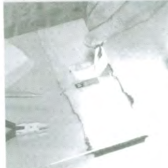
5. Spreading the adhesive
