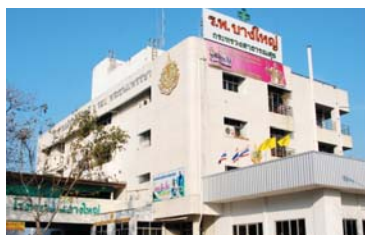
Bangyai hospital : a 30 bedded hospital
