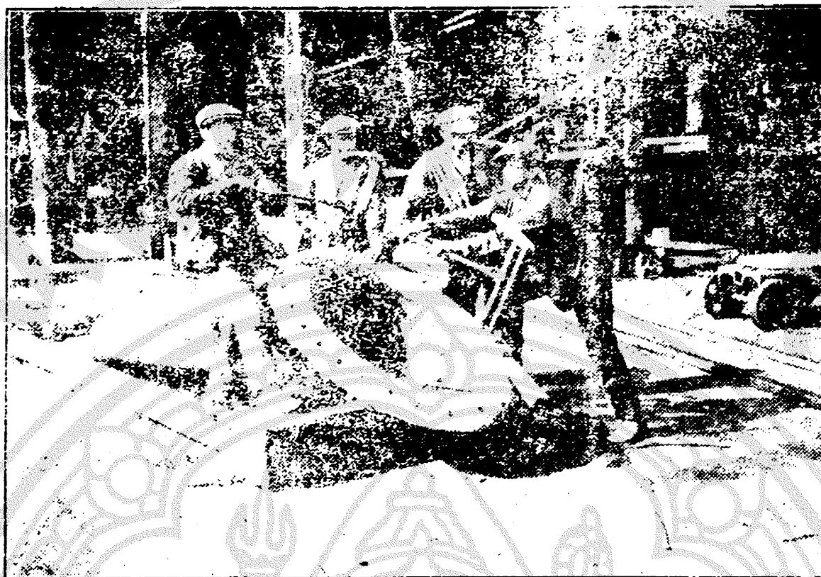
WITH THE BRITISH NAVY IN WAR TIME. STANDARD SHIP'S IN VARIOUS STAGES OF CONSTRUCTION. Preparing a hawse pipe.
