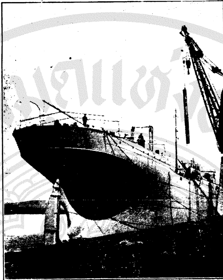
OFFICIAL PHOTOGRAPH WITH THE BRITISH NAVY IN WAR TIME Standard ships in various stages of construction. Finishing off. Lowering a ventilating shaft into the ship.
